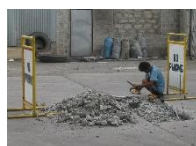
Road under repair:
